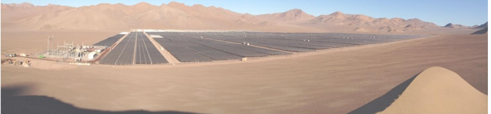
General view of the “Amanecer Solar” Plant site, as of March 2014
